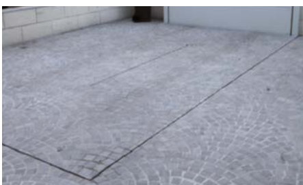
Synthetic stone covering (3 cm thick)
